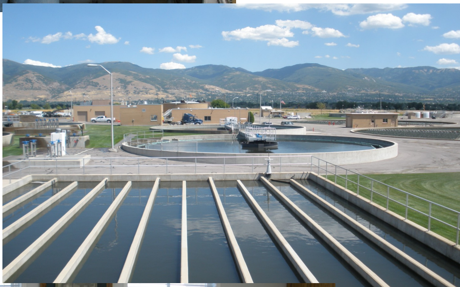
North Plant— Secondary Clarifiers & Chlorine Contact Basins
