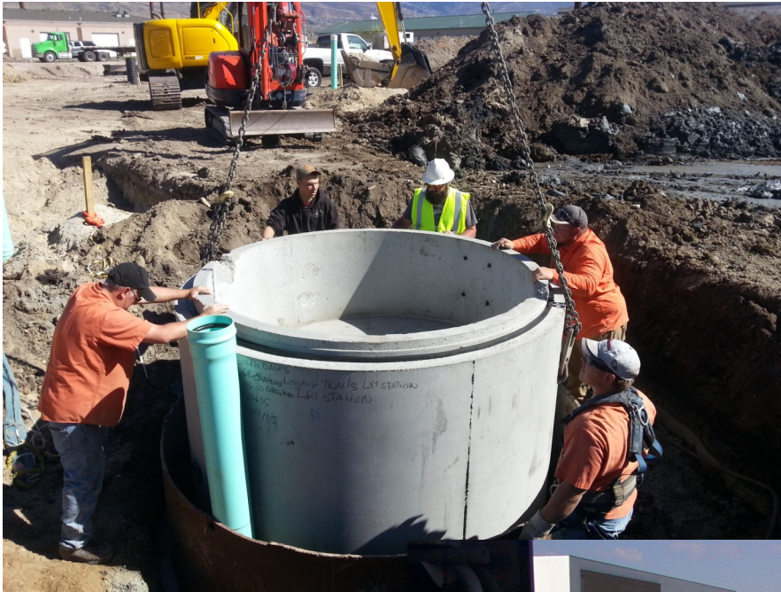
Construction of Legacy Trail Lift Station
